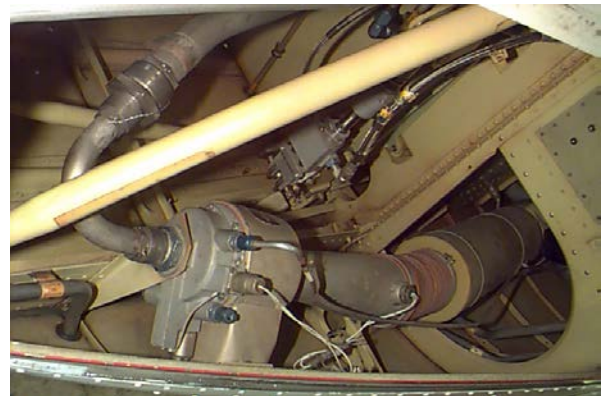
Figure 12-2 Tail Rotor Servoactuator in Heater Compartment
